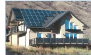
Figure 1 South-facing rooftop PV array and balcony PV array of the Green Dream Home
